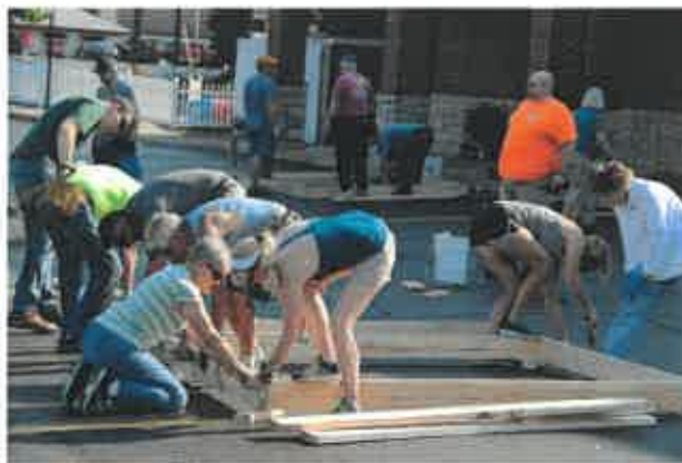
Catching the Building Spirit Habitat for Humanity Build
